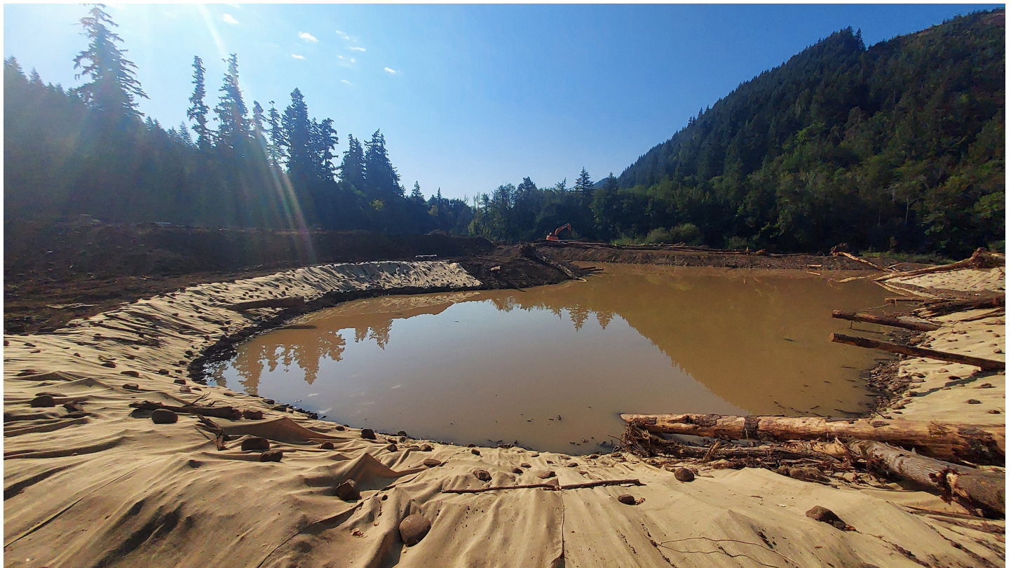
Burlap will help to control erosion until new plantings are well established
