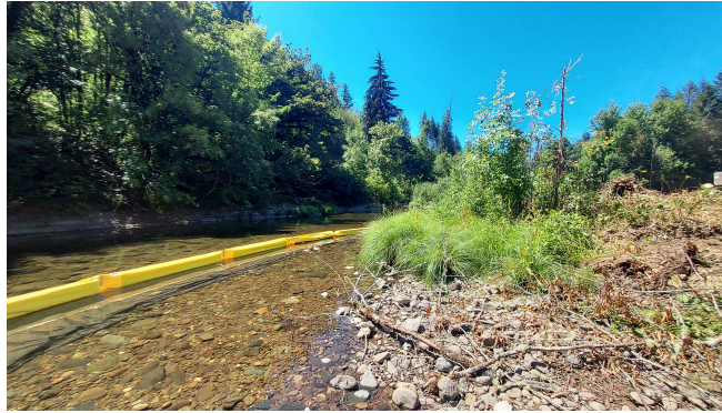
Silt curtains installed in Mosby Creek at the work site.
